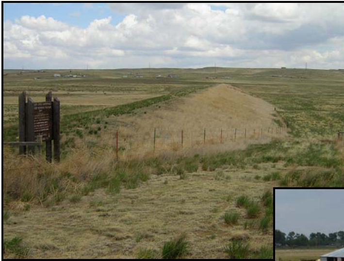
Boxelder B-4 embankment
